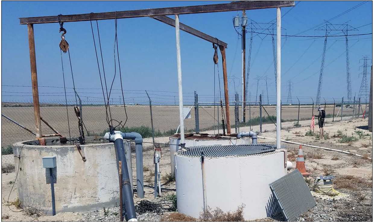
Standpipe cluster constructed between 1956 and 1967; view to the northwest
