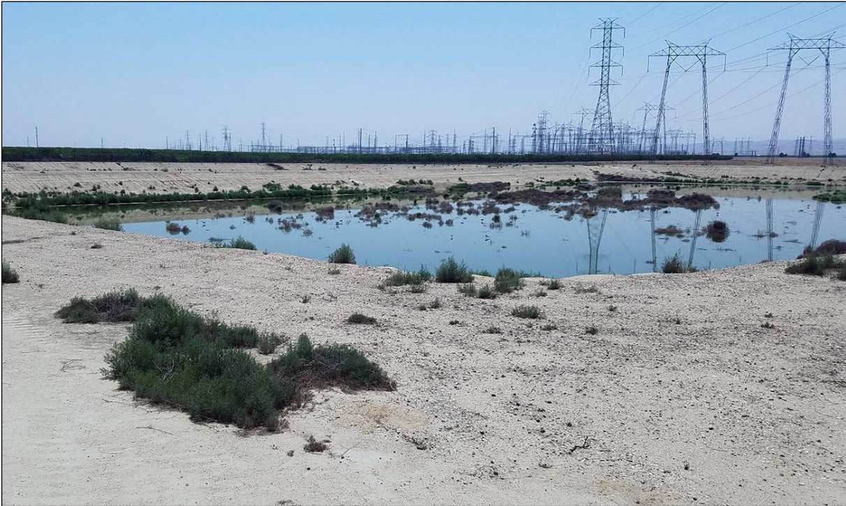
Modern 22.5-acre-foot storage pond; view to the southeast
