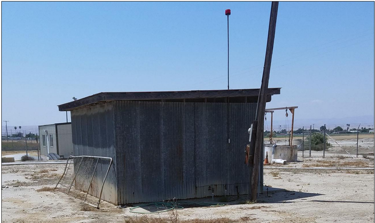
Electrical shed constructed between 1956 and 1967; view to the southwest
