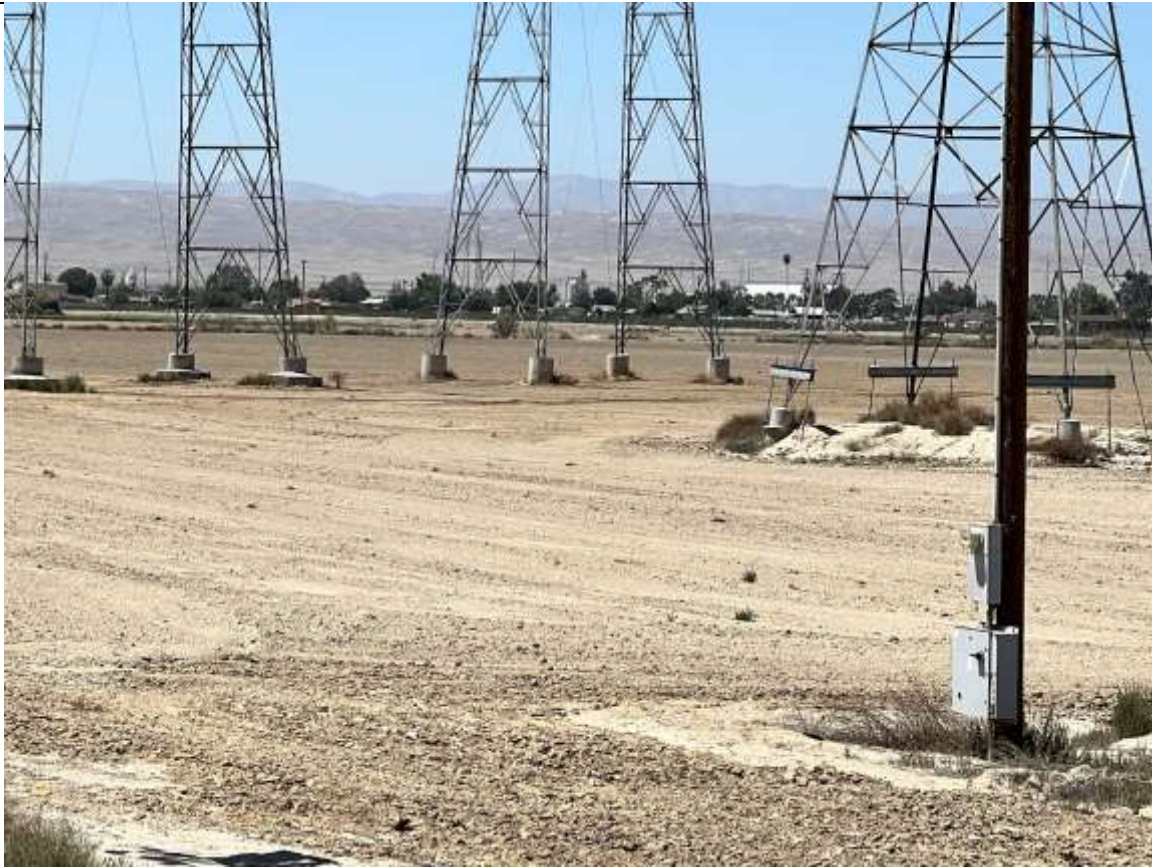
Photo 4. Looking N at proposed WWTP.
