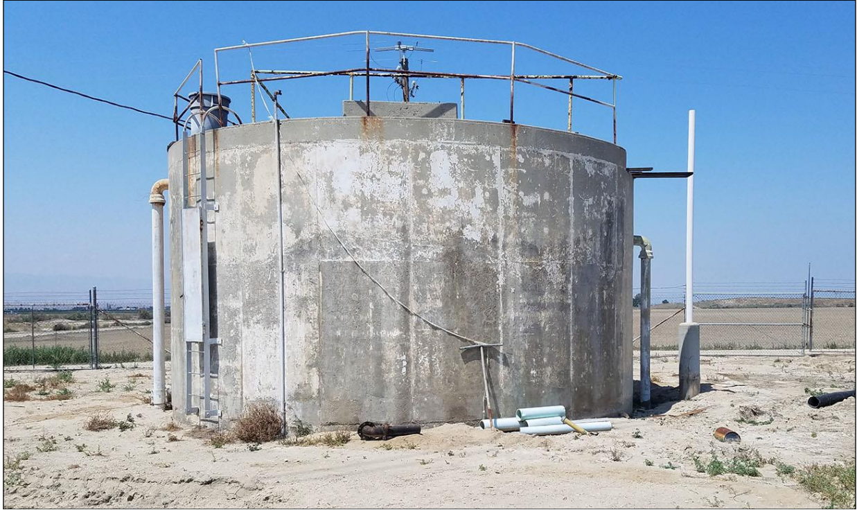
Imhoff tank constructed between 1956 and 1967; view to the west
