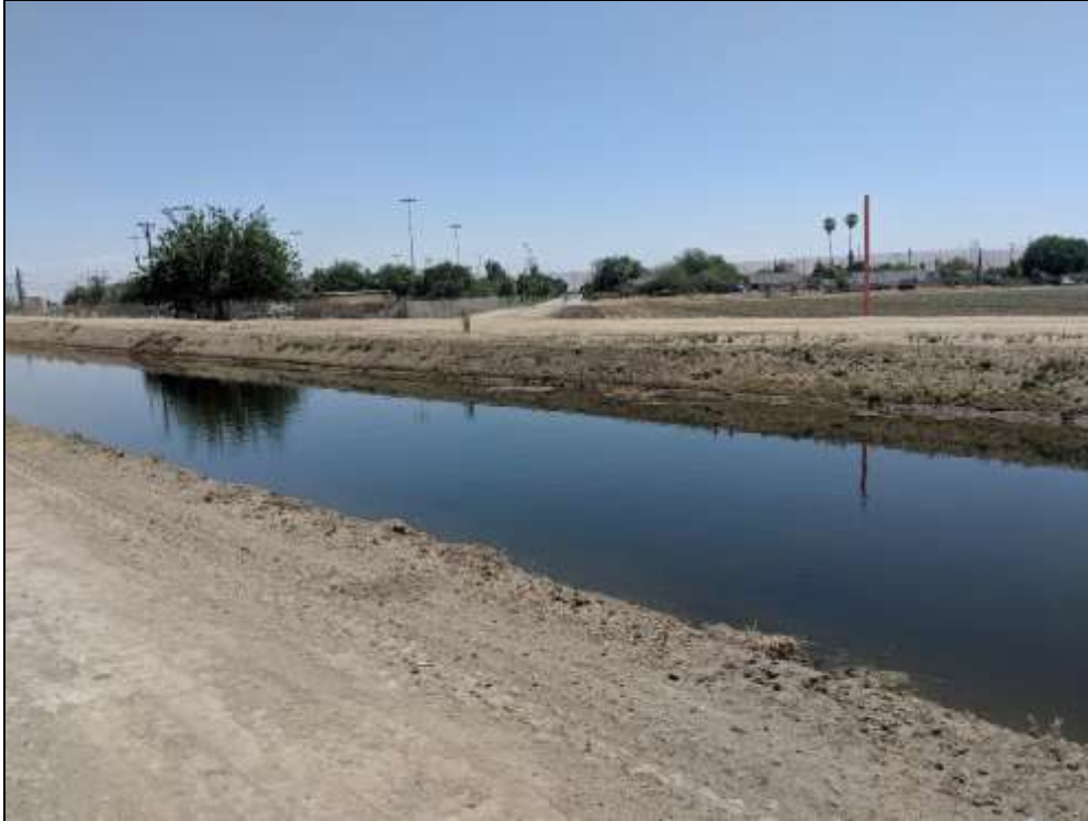
Photo 3. Canal that will be crossed by the associated potable water pipeline.
